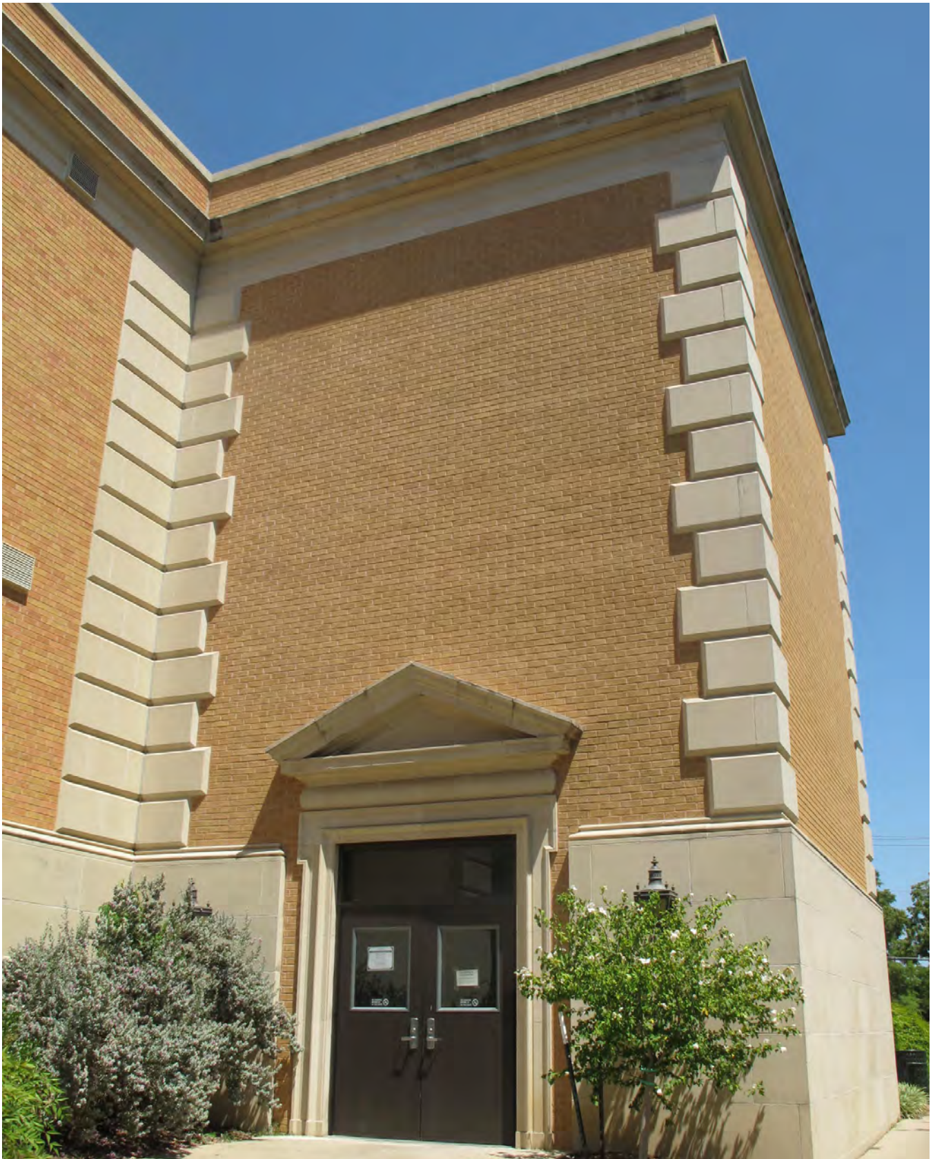
Above is an example of an appropriate expression of the building base, with rusticated quoins terminating fields of brick and defining the building corners; the cornice and extended parapet are seen on many campus buildings. The doorway is given depth and expression with stone trim and pediment.
