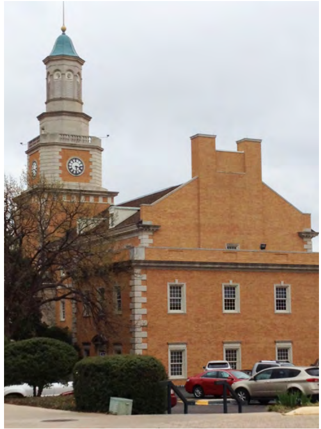
Hurley Administration Building creates an interesting roof profile against the sky with a sloped roof, dormers and an expressive end wall.
