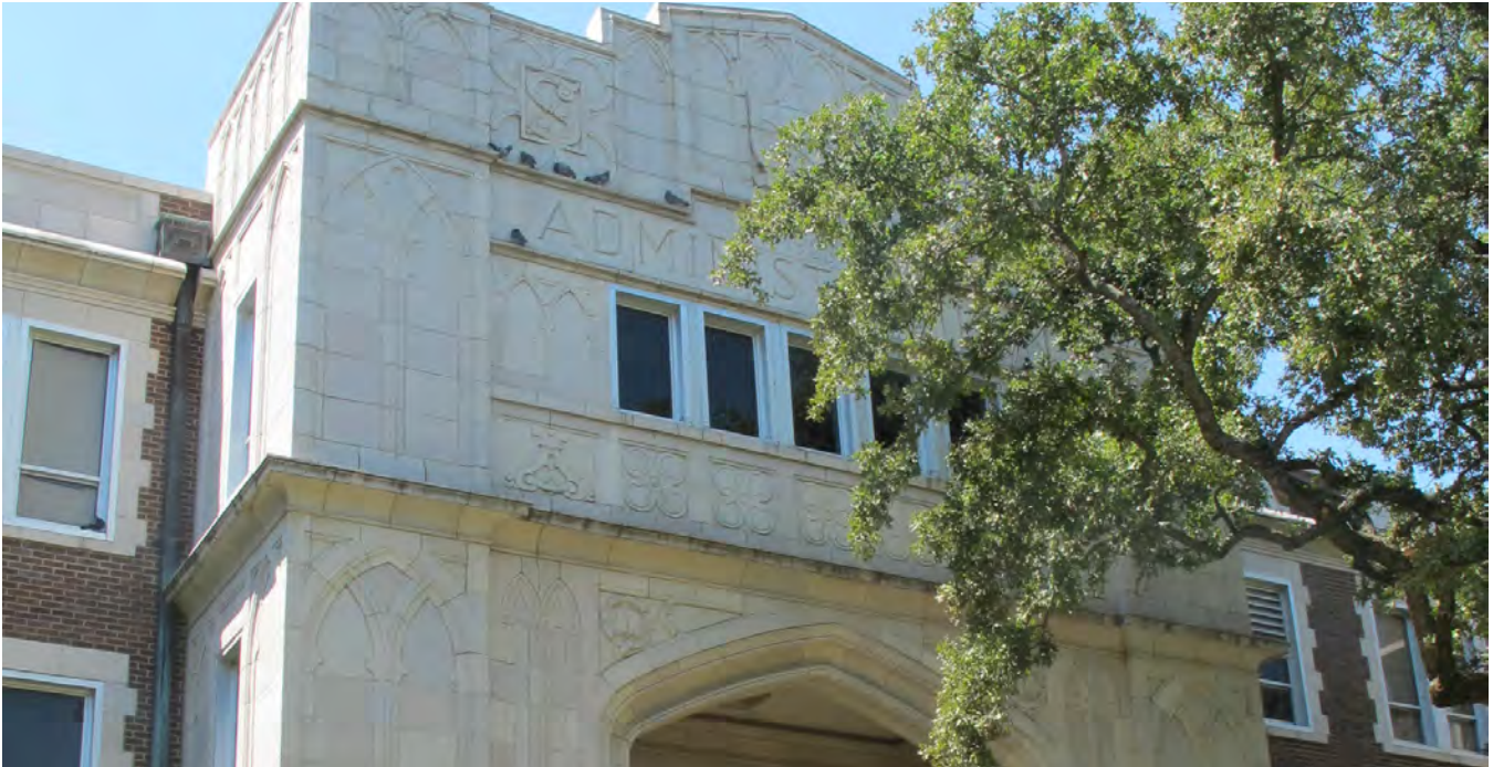
Stone should be used as a decorative accent material, especially at main entrances, as seen at the entrance to the Auditorium Building above.
