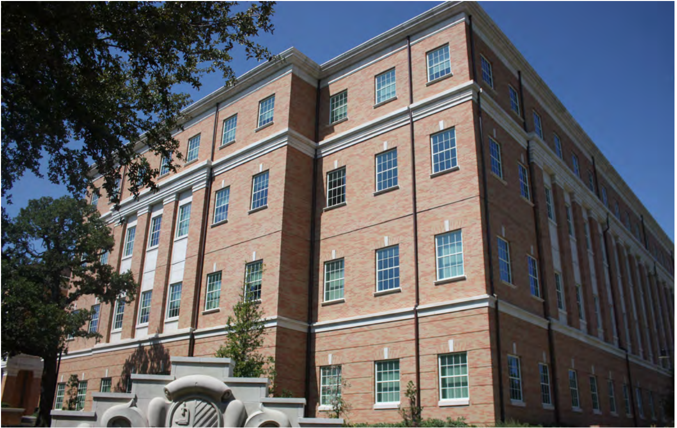
Life Sciences expansion is an energy-efficient facade with a strong base, middle and top. Note the vertical expression given to the middle section; details include stone string courses delineating each section and lintels with keystones, except on the top level which is differentiated by simpler windows.
