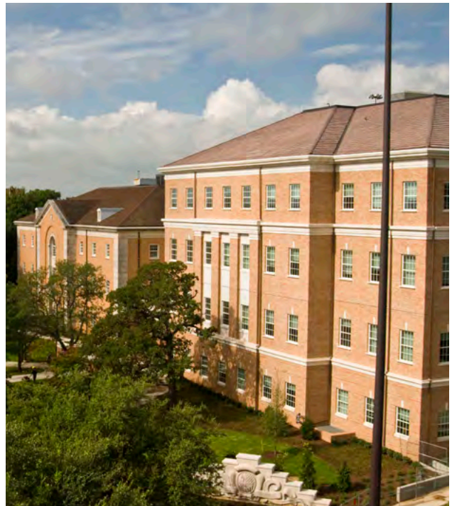
Life Sciences Building hipped roof with cornice edge.
