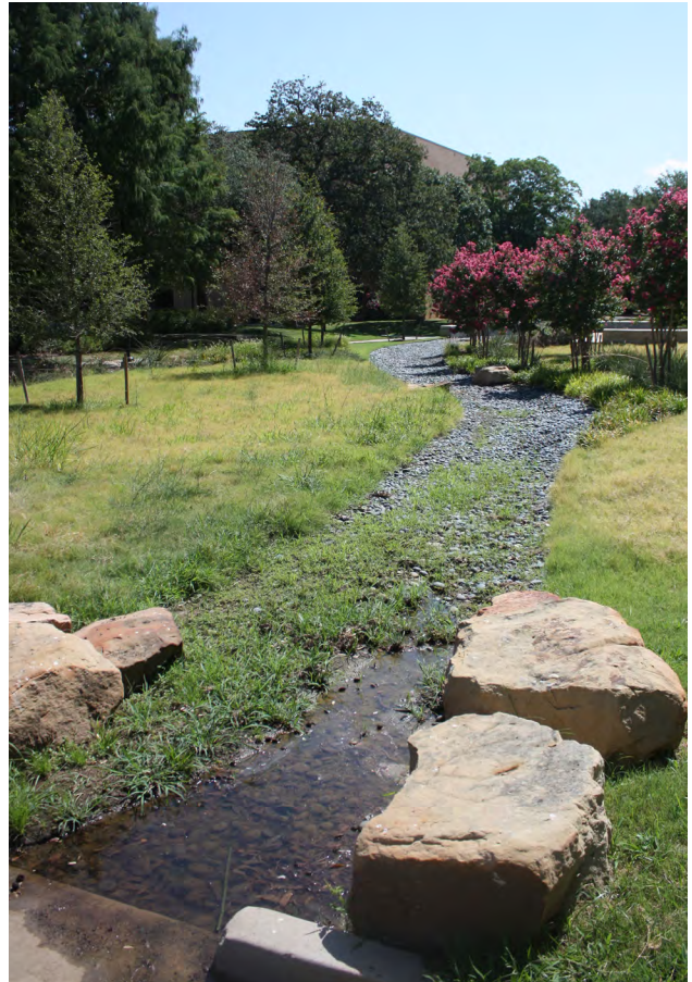
Above and below are images of the project at the east end of Sycamore; hardscape and landscape blends with storm water management to create an inviting place, recapture run-off and eliminate mall flooding.
