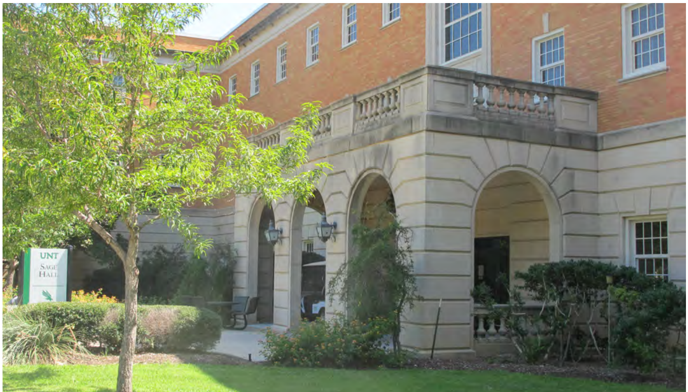
Sage Hall exhibits a well-proportioned stone entry portico providing a comfortable entry transition
