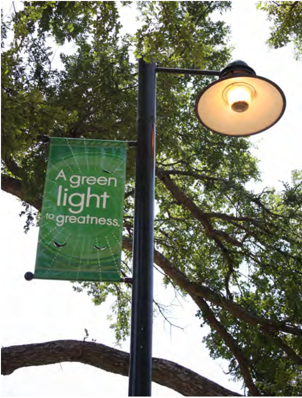
UNT standard pedestrian-oriented lighting with banner arms should be used on all campus streets and pedestrian malls and should be added to perimeter streets to reinforce the campus identity.
