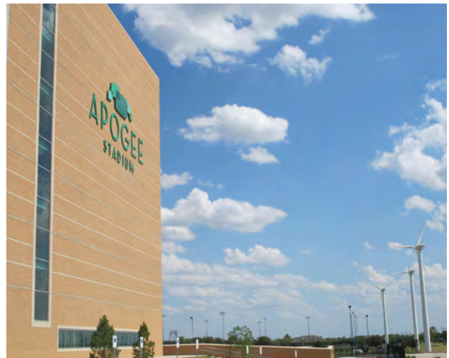
Stadium identity along I-35 from the north approach to campus
