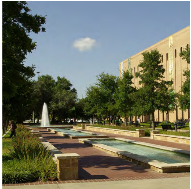
Completed Library Mall project.
